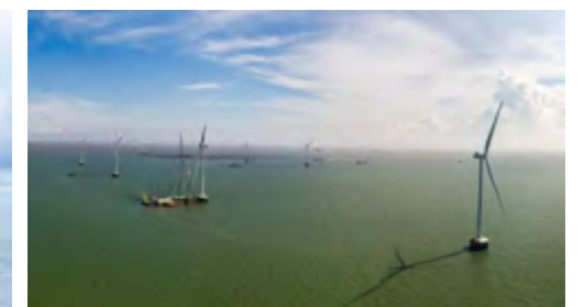
Vietnam Tra Vinh II 48MW Offshore Wind Farm Project
